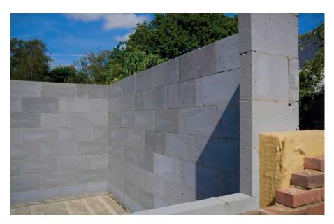
The Thin-Joint, Rå Build method of construction enables a fast, weathertight masonry shell to be built, allowing follow-on trades to start work sooner in a weatherproof environment, whilst retaining the flexibility of on-site construction. Thin-Joint is a recognised Modern Method of Construction and has been fully adopted as the preferred method of wall construction throughout most of northern Europe.
